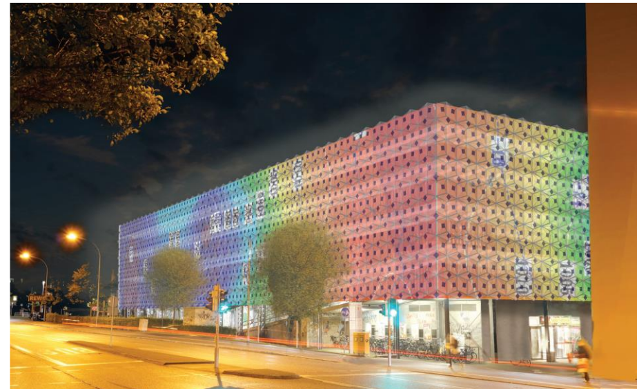
Example of Use – the Future Solar Garage Vauban, Freiburg, Germany
